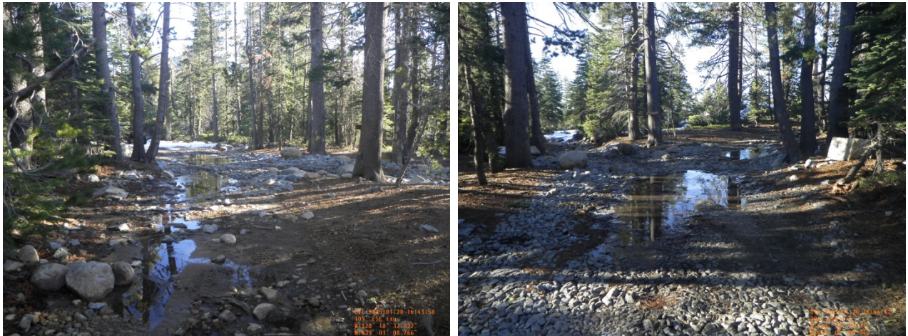
Ellis Creek Intertie RT Station 99+86
