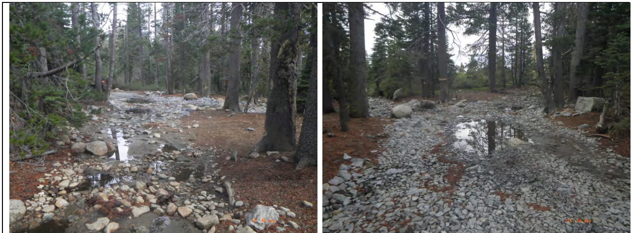
Ellis Creek Intertie RT Station 99+86
