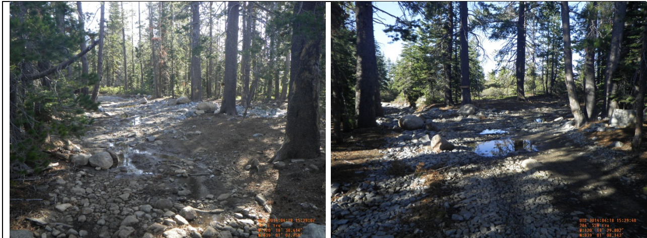
Ellis Creek Intertie RT Station 99+86.95
