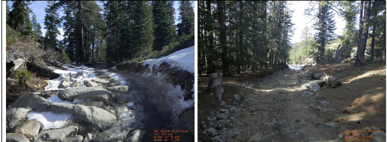
Walker Hill RT Station 170+80
