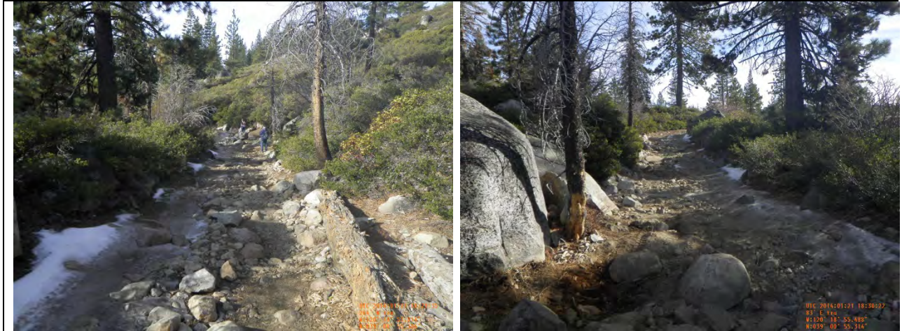
Post Pile RT Station 75+00
