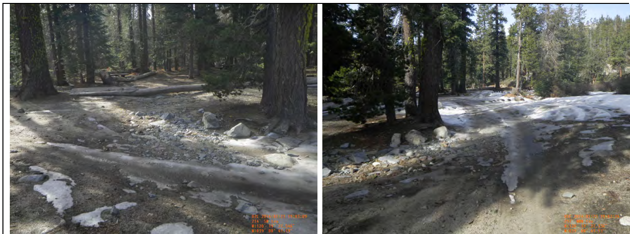
Wentworth Springs Campground RT Station 33+65.67
