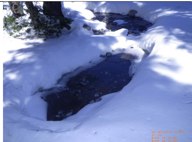
Wentworth Springs Camp Ground RT Station 33+65.67 Water Depth: 0.2' The Rock Ditch Crossing (RDX) was exposed through the snow, with run off moving across the RDX. The water was clear with no signs of sediment moving in the water.
