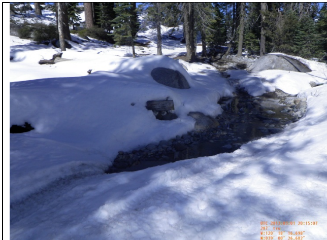
Gate Keeper LL Station 146+77.03 Water Depth: 0.4' The Rock Outlet Protection (ROP) was exposed through the snow, with run off moving across the ROP. The water was clear with no signs of sediment moving in the water with the flow appearing to be moving towards the snow covered BMP.
