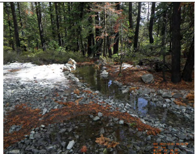
Rock Energy Dissipater RT Station 99+86.95
