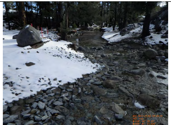
Rock Breast Wall RT Station 209+58.39
