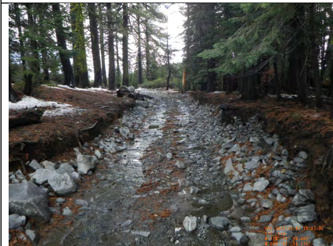
Rock Fill RT Station 170+00
