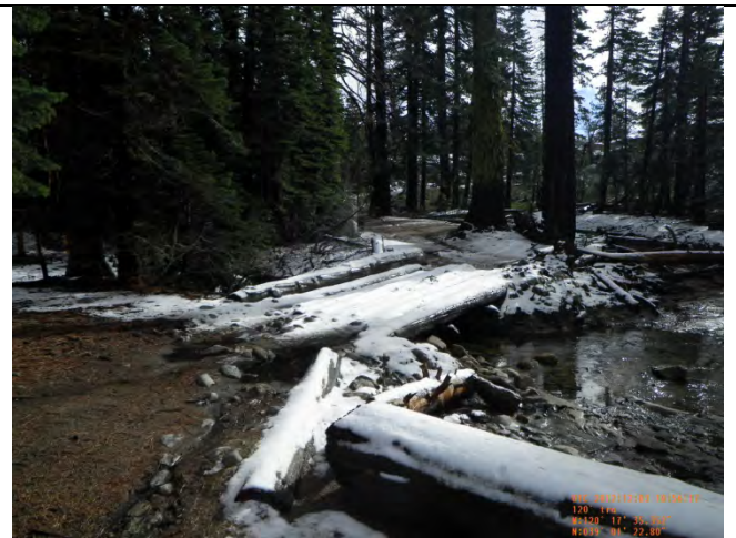
Log Bridge RT 155+48
