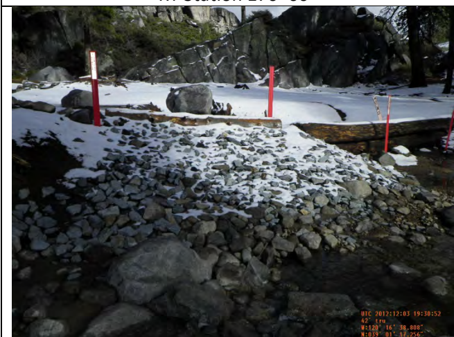
Rock Fill RT Station 209+58.39
