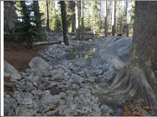
Rock Fill LL Station 147+44.50
