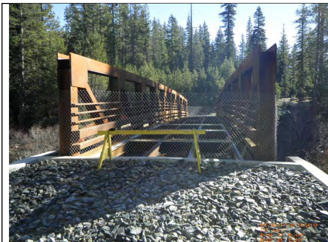
Gerle Creek Bridge
