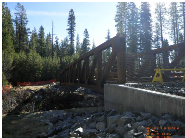
Gerle Creek Bridge
