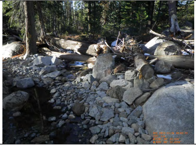
Rock Outlet Protection LL Station 148+75.49
