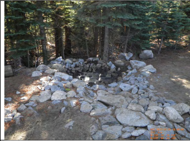
Rock Energy Dissipater LL Station 148+75.49
