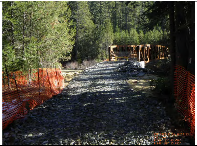
Gerle Creek Bridge
