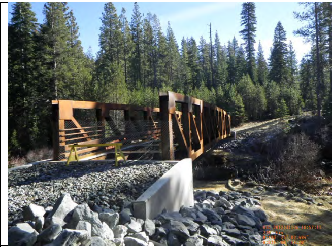
Gerle Creek Bridge
