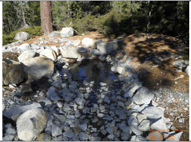
Rock Ditch Crossing LL Station 148+75.49
