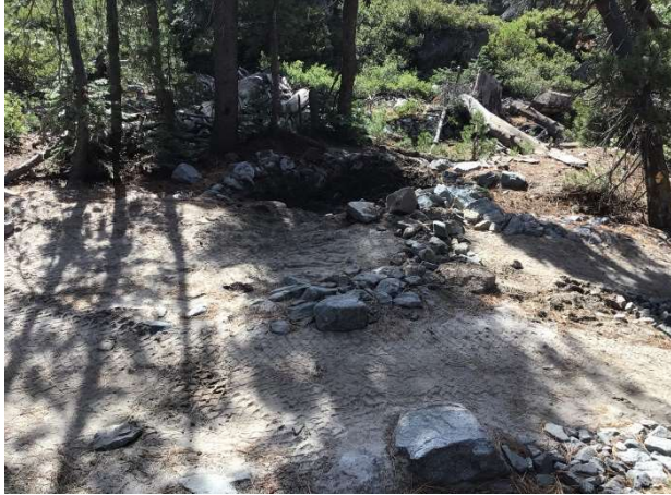
Photo of BMP work in progress
