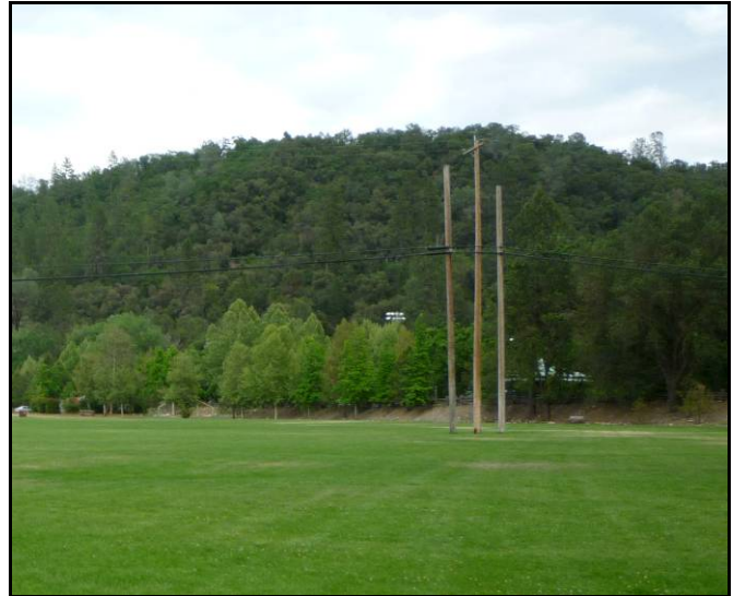
Utility poles in multiuse field at HLP
