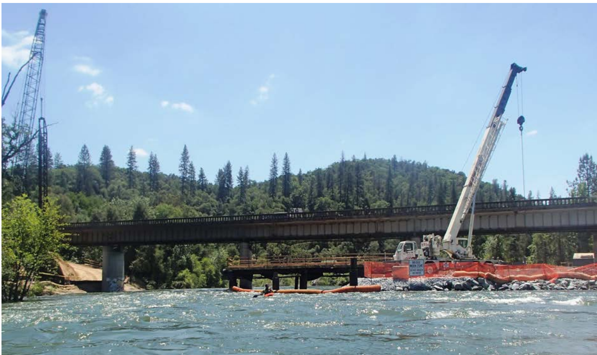
Photo 6. Hwy 49 Replacement Bridge construction
