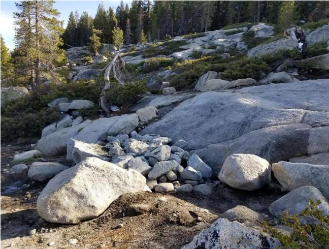
Indian Bypass-Rock was added to assist with the drop off and protect the soils
