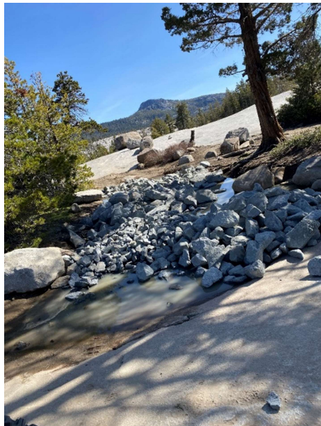
Hole at the top of Hot Rock to armor the soils.
