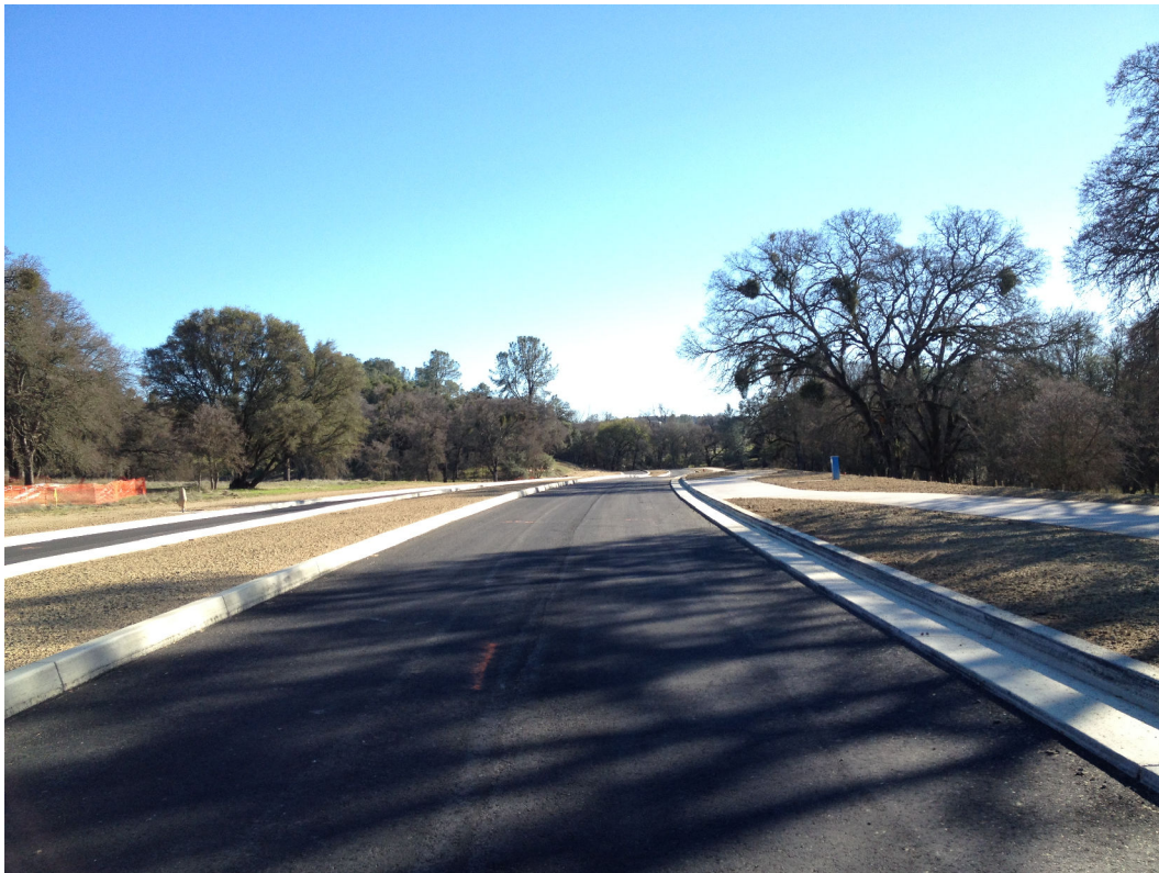
Figure 3.2-2(d): View from Silver Springs Parkway North Segment Facing South
