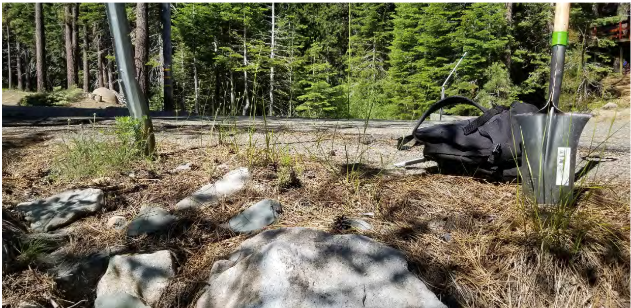
Photo 10: Culvert 3, C3, looking northwest (upstream).
