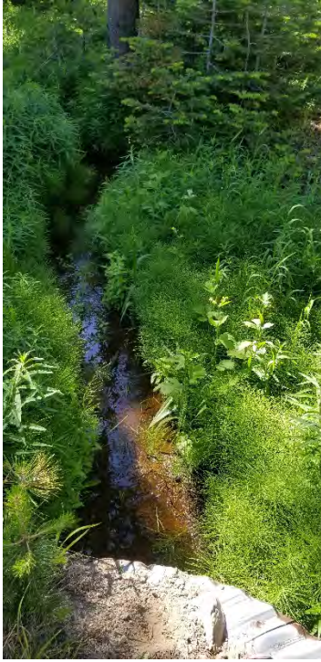
Photo 7: Culvert 2, C2, looking southeast (downstream).
