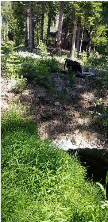
Photo 8: Culvert 2, C2, looking northwest (upstream).
