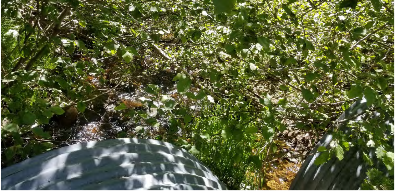
Photo 9: Culvert 3, C3, looking southeast (downstream).
