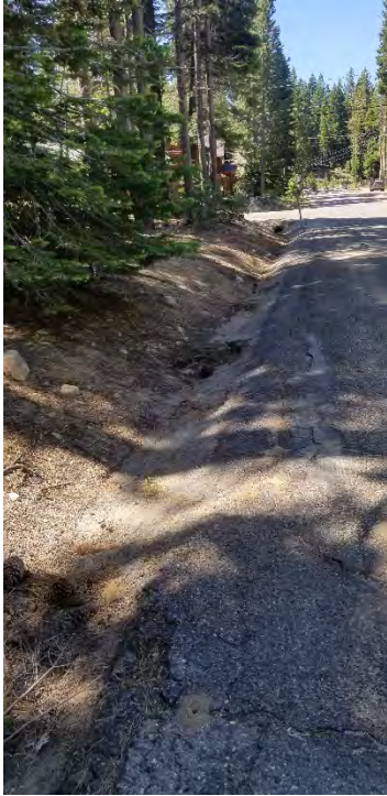
Photo 11: Culvert 5, C5, Roadside ditch (non-jurisdictional), looking west up San Bernardino road.
