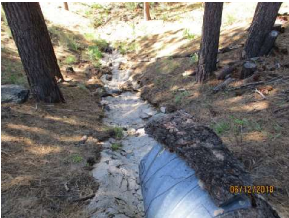
Photo 6: Unnamed Drainage 2, Data Point OHWM 2, looking downstream at culvert.
