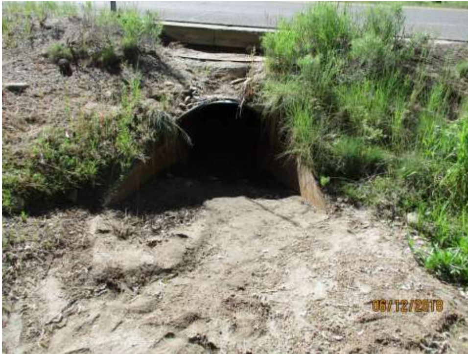
Photo 1: Unnamed Drainage 1, Data Point OHWM 1, looking upstream at culvert.
