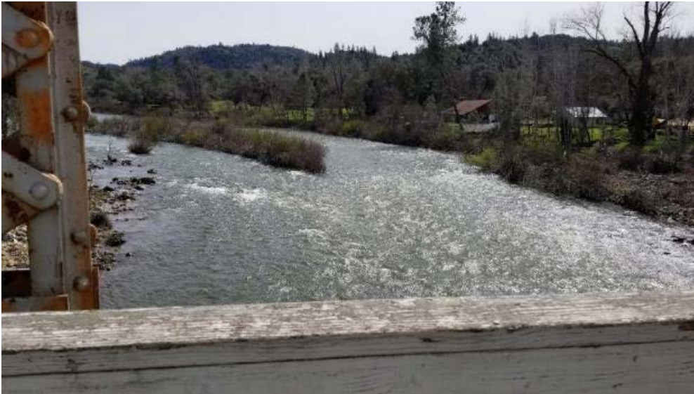
Figure 3-10. KOP 5 Existing Condition
