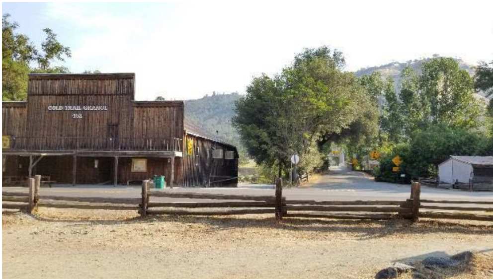
Figure 3-2. KOP 1 Existing Condition
