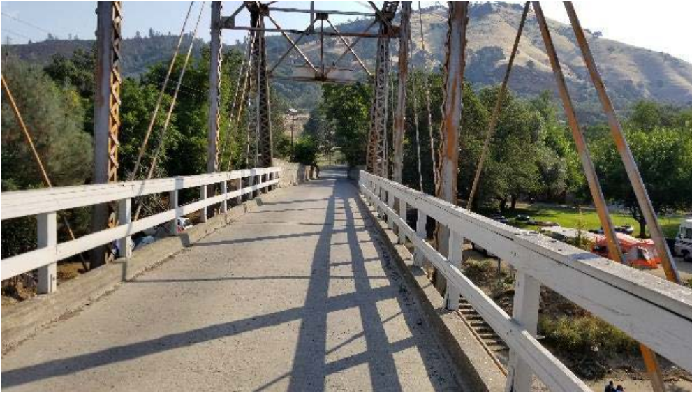
Figure 3-4. KOP 2: Existing Condition
