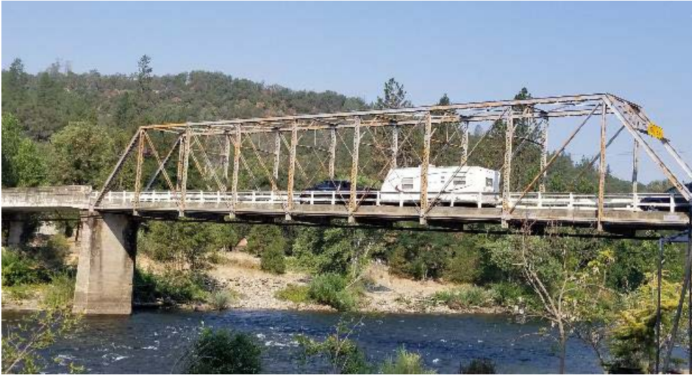
Figure 3-8. KOP 4 Existing condition
