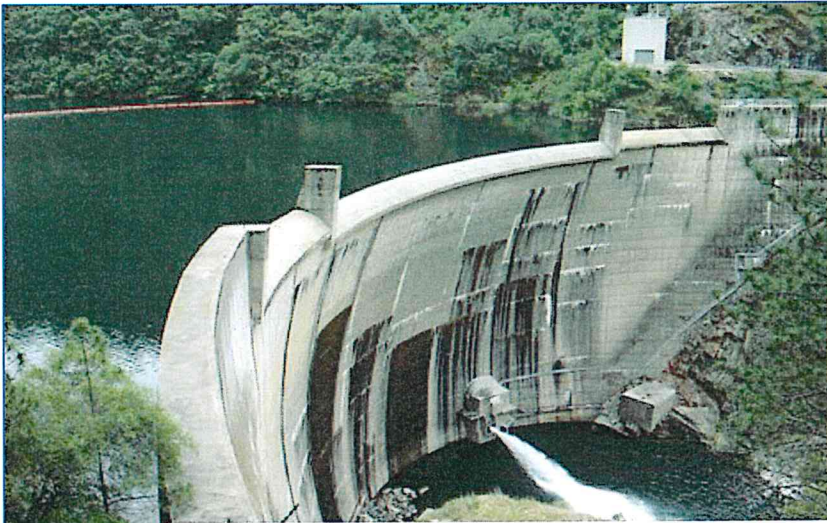
Photo 7: Slab Creek Reservoir 3.5 miles above Mosquito Bridge
