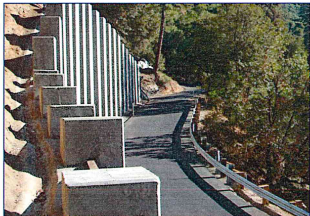
Soldier Pile Wall Constructed in 2007
