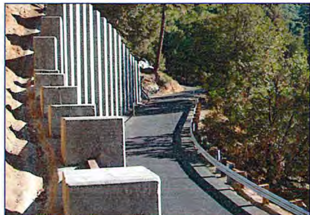
Soldier Pile Wall Constructed in 2007
