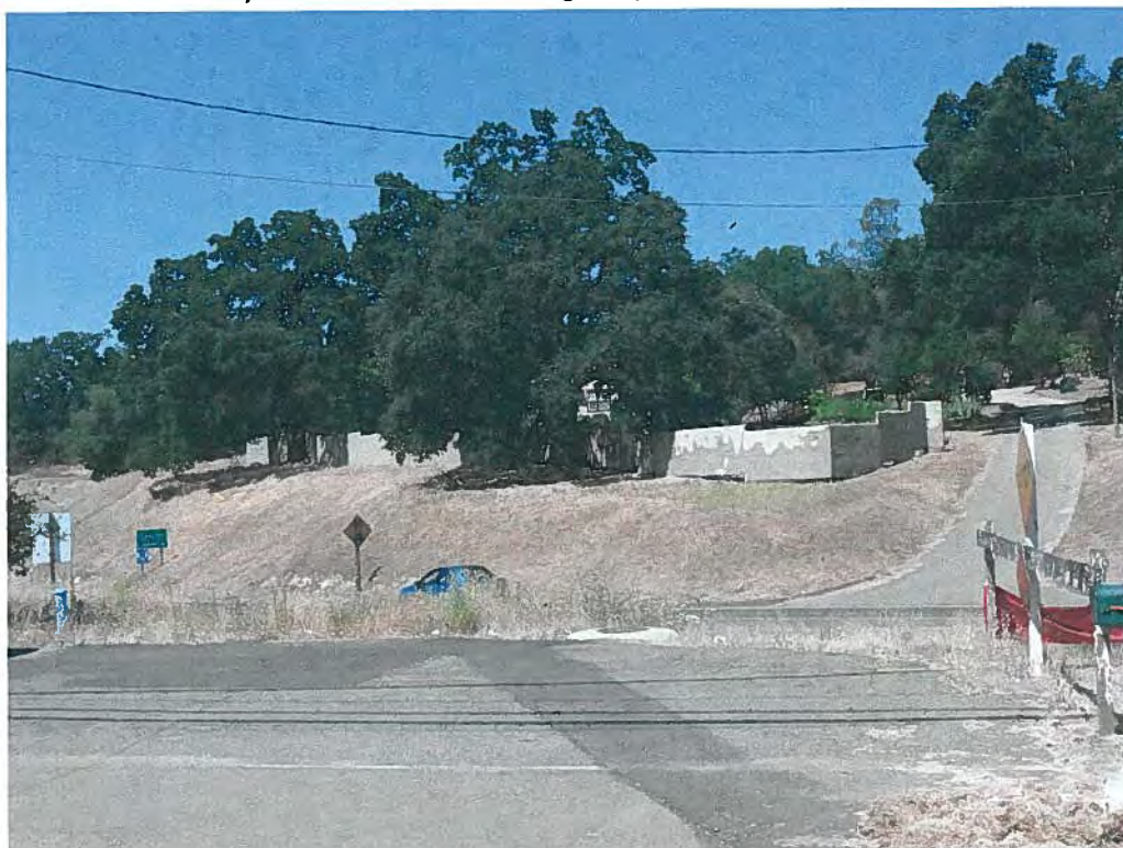
Picture 14: Privacy wall above widened Highway 49
