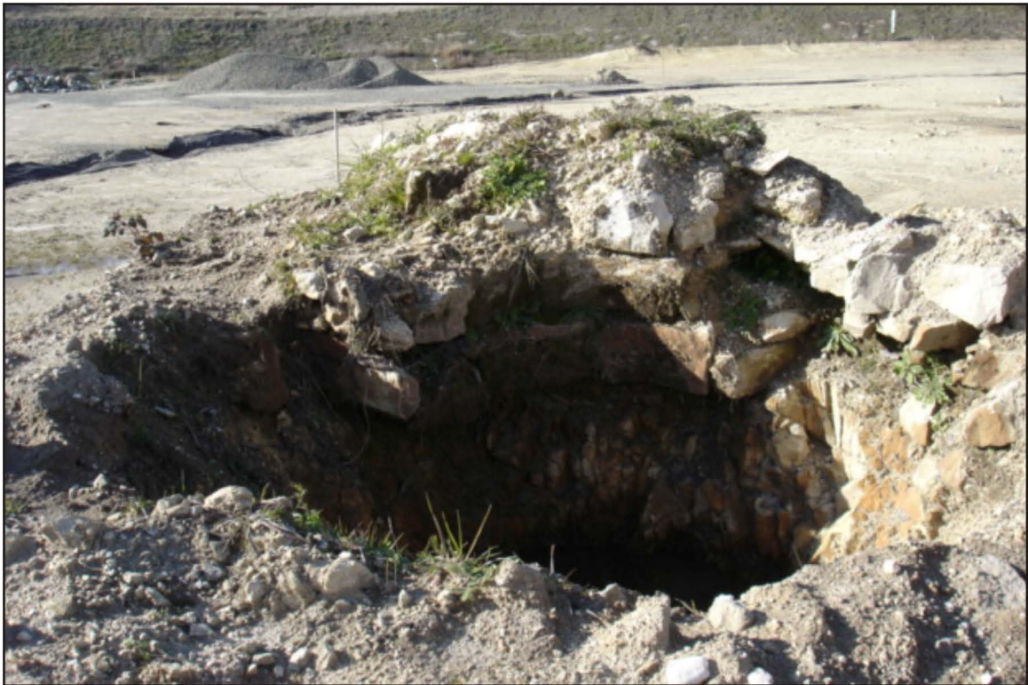
Photograph 4: P-9-1825. Facing west.
