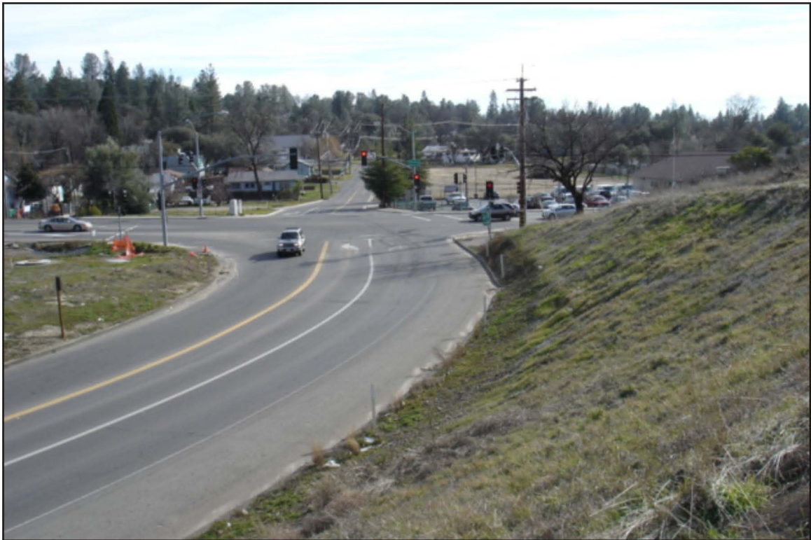
Photograph 2: P-9-1149. Facing south.
