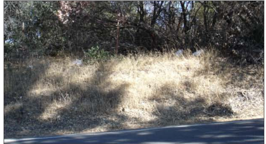
Photograph 4: Vertical rise along eastern side of SR-49.
