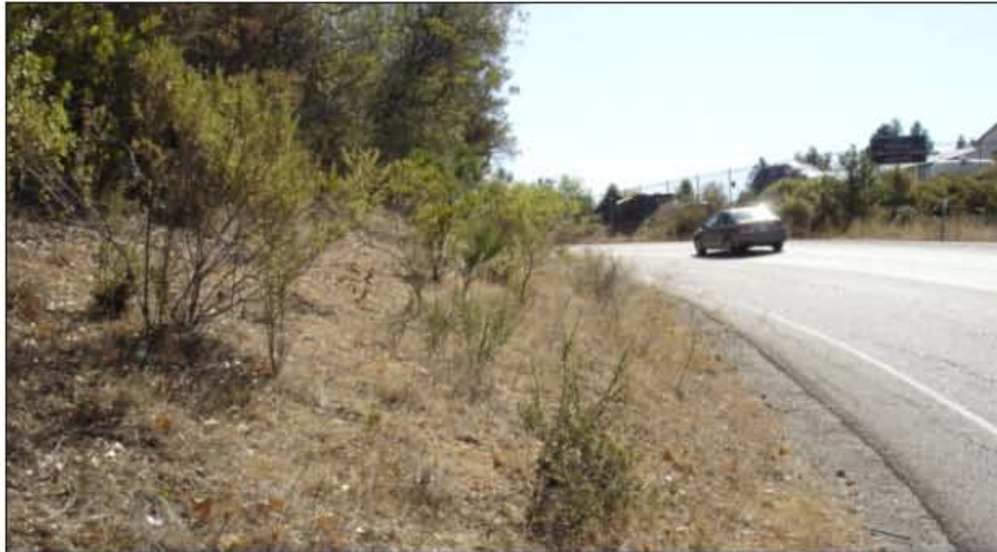
Photograph 3: Illustrates narrow shoulder along eastern portion of SR-49.
