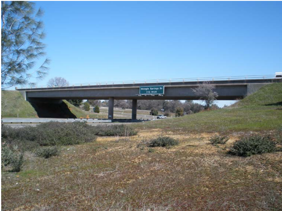
Existing Ponderosa Overcrossing
