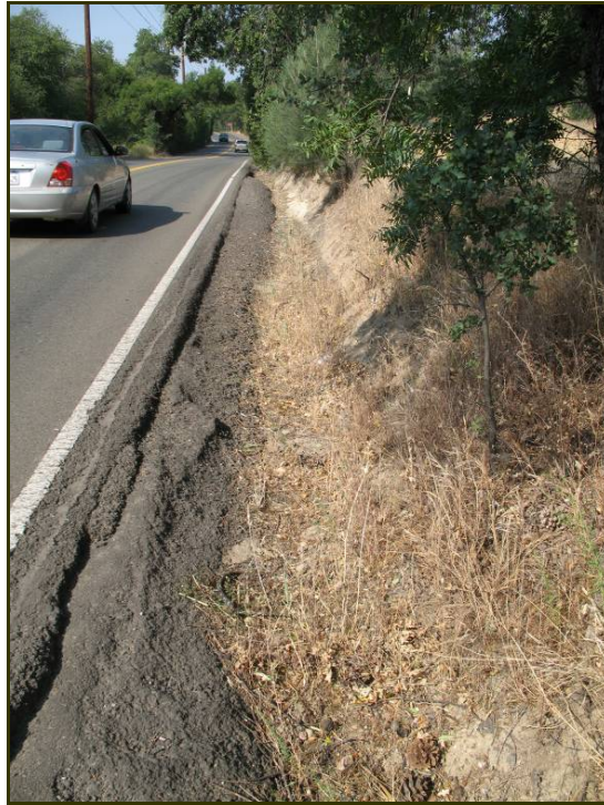
Photograph 3. Photograph of roadside ditch (RD1) located on the north side of Pleasant Valley Road near the northern end of the study area. Photograph taken from the eastern end of the ditch looking southwest along Pleasant Valley Road.
