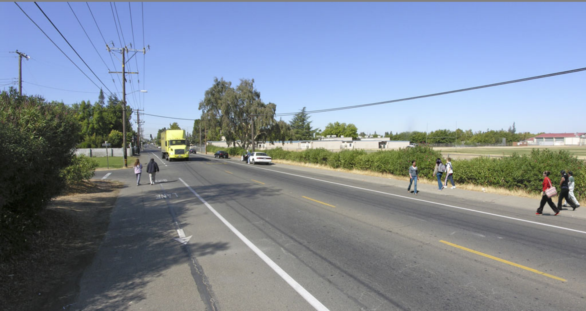
At another, more rural section of Hurley Way, pedestrians lacking sidewalks walk in bike lanes.
