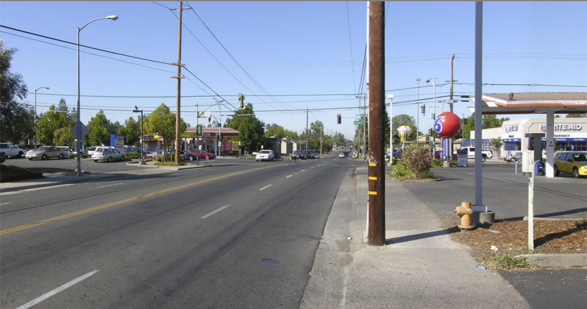
The original photo of the intersection of Hurley Way and Fulton Avenue, east of downtown Sacramento, shows a narrow sidewalk, street-front parking lots, poorly marked crosswalks and no protection from the sun.
